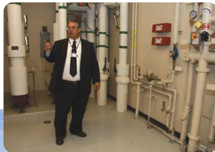
Duane Devey, energy supervisor, Jordan School District, shows the pipes of the ground-source heating system.
