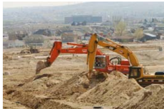
Crews work on the Daybreak development.
